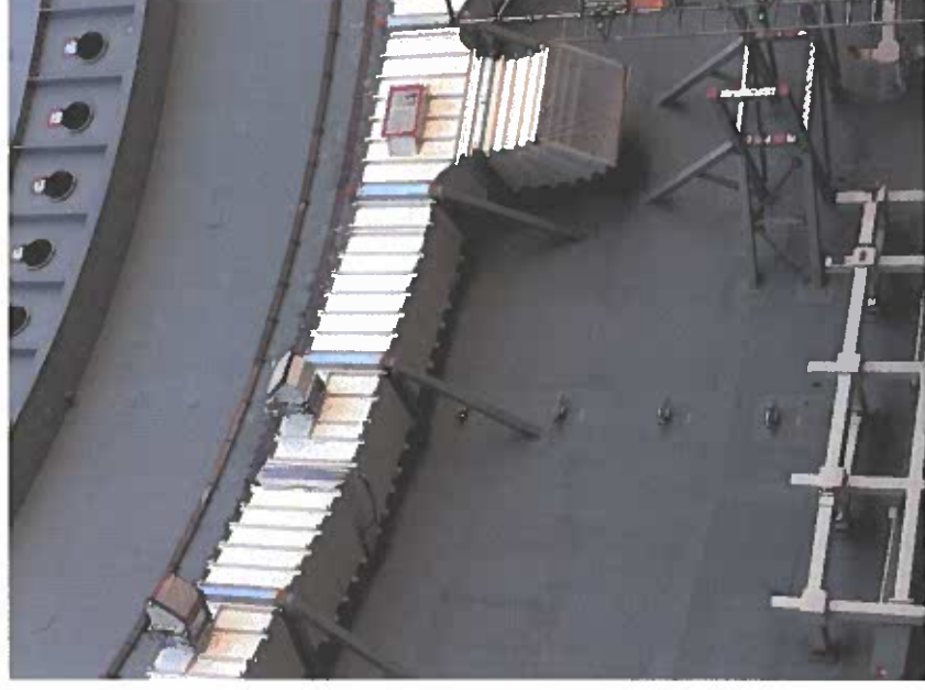
Unit 2 Containment – Coated and Sealed
