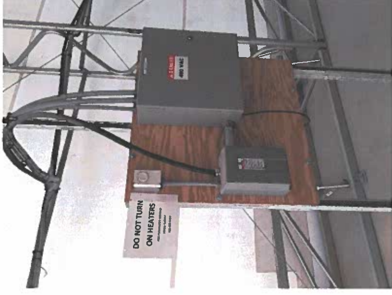
Heaters in place in tents
