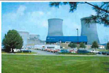
Watts Bar Unit 2 Completion (2007 to present)
